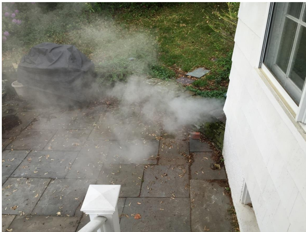
Figure 25: Condensate from a Condensing Boiler
